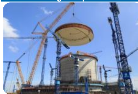
Fangchenggang Unit 3 Dome Lifting Completed
